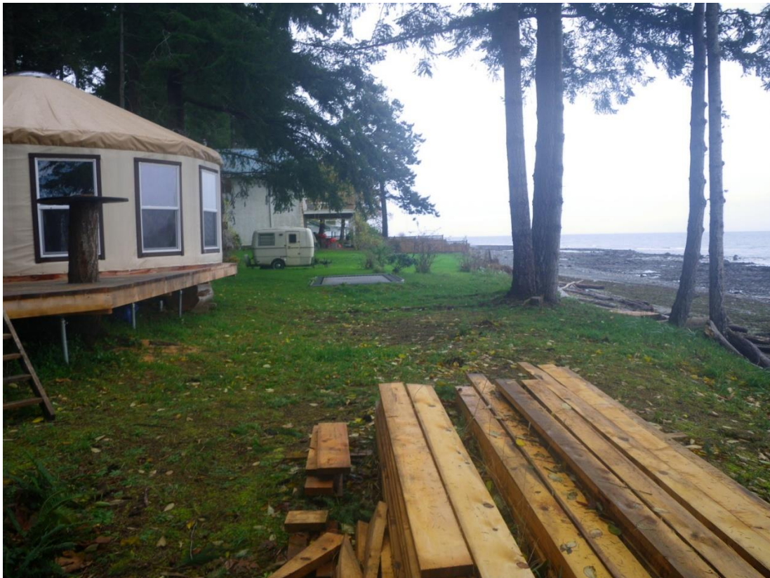
Figure 2: Deck Exceeding 600mm to the Adjacent Ground
